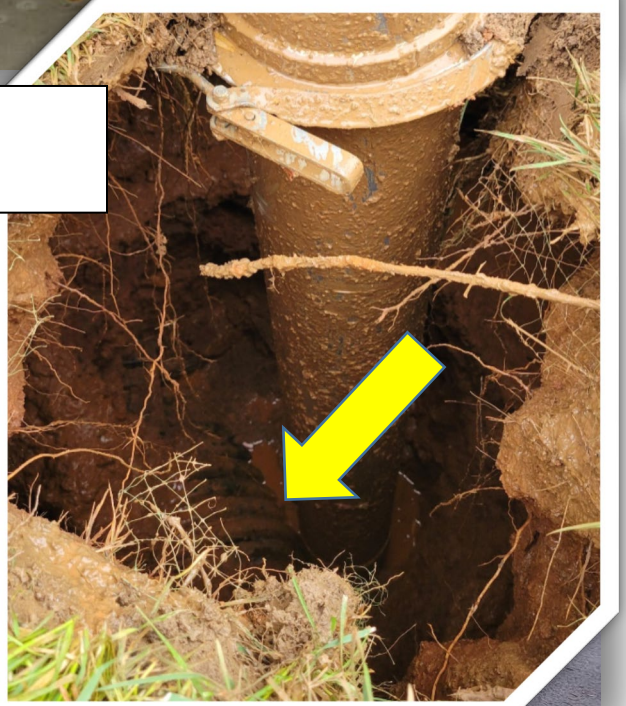
Stormwater Infrastructure failure created sinkhole (9 December)
