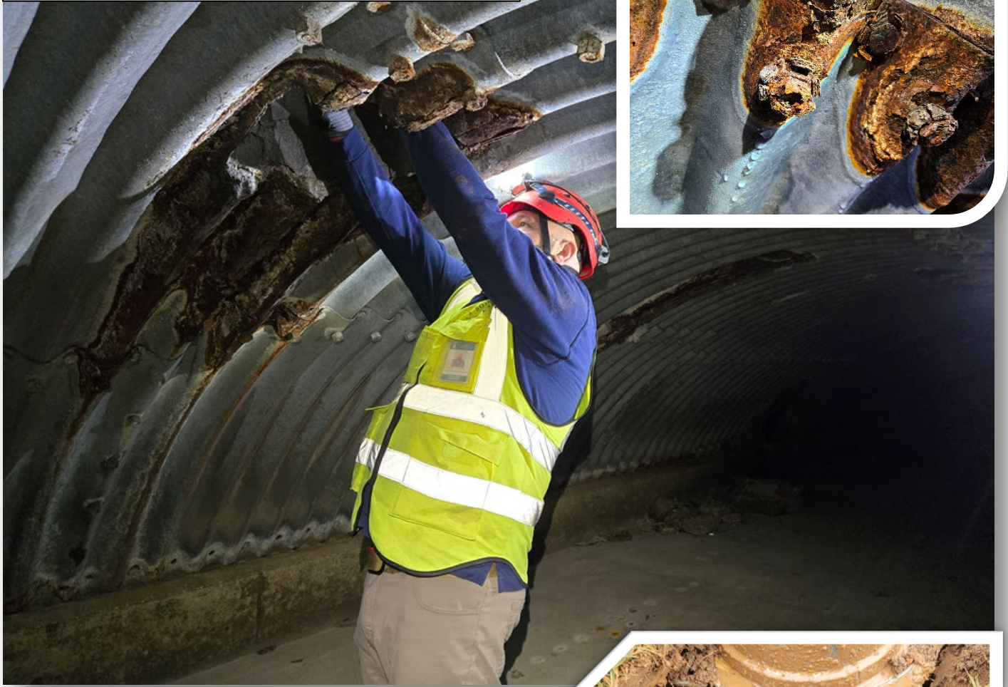
Stormwater Infrastructure failure created sinkhole (9 December)
