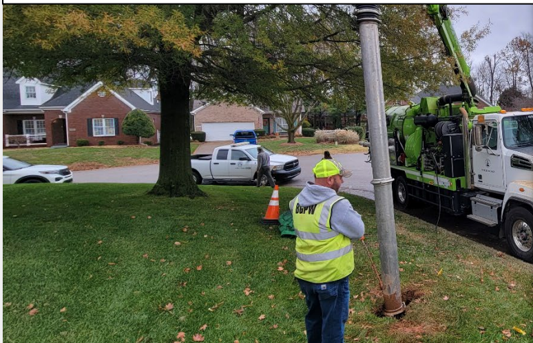
Stormwater Infrastructure failure created sinkhole (9 December)
