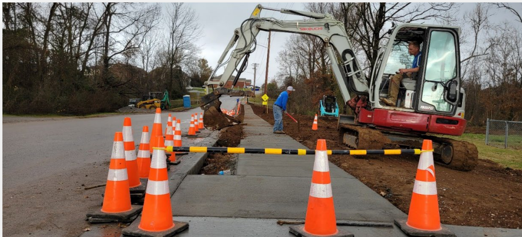
Figure 6-Final construction of the new sidewalk on Creekwood Avenue (09 December)
