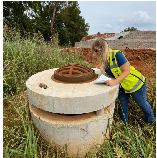
Figure 4-Construction Coordinator I Dara Price inspects a water quality unit at Cherry Farms Apartments (16 July)
