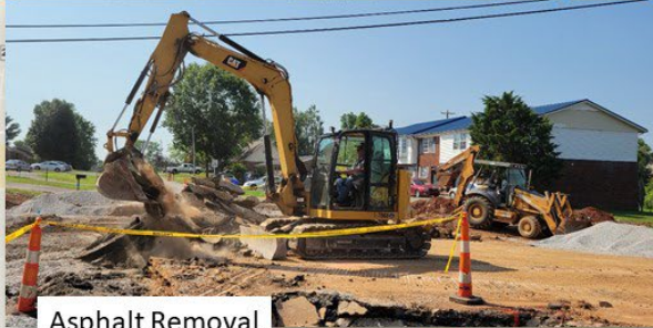
Asphalt Removal
