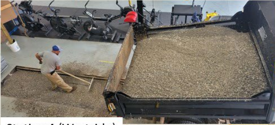
Station 4 (Westside) Rock Filling
