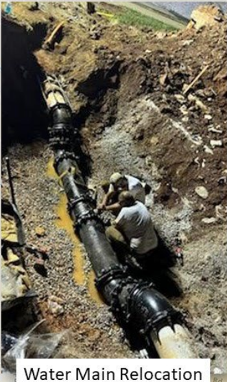
Water Main Relocation
