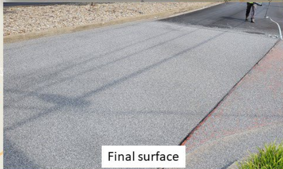
Epoxy applied over the "friction" aggregate
