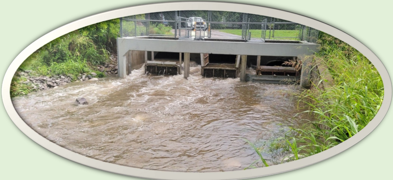
Figure 1- During heavy rains, the Environmental Compliance Division inspects critical stormwater infrastructure. This photo shows the Whiskey Run water quality unit during the 17-18 July storms.
