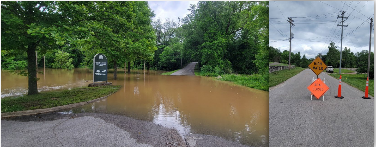
Figure 4-Operations crews closed Boatlanding Road and placed warning signs to inform the public due to flooding. The city also updated social media content to help maximize communications. (10 May)
