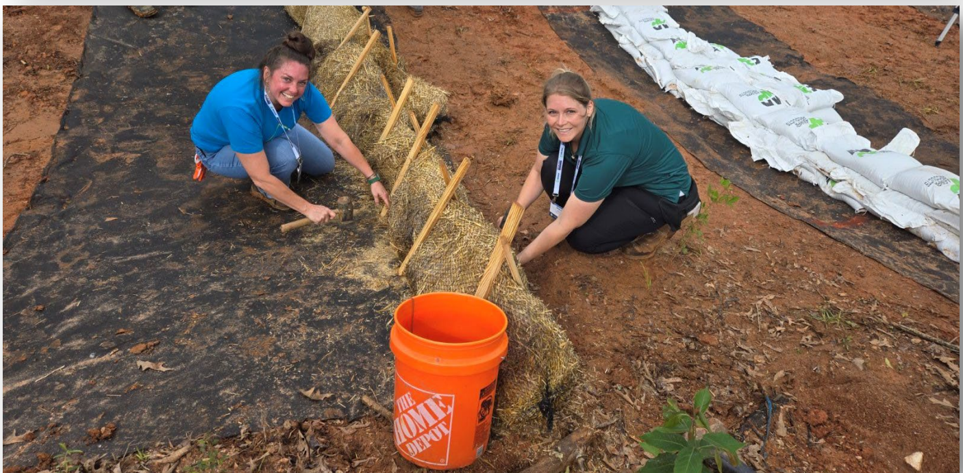
Figure 8-Environmental Compliance Inspector Courtenay Howell (left) and Construction Coordinator I Dara Price (right) practice Erosion Prevention and Sediment Control techniques in the field during training at Auburn University in Alabama. (14 May)
