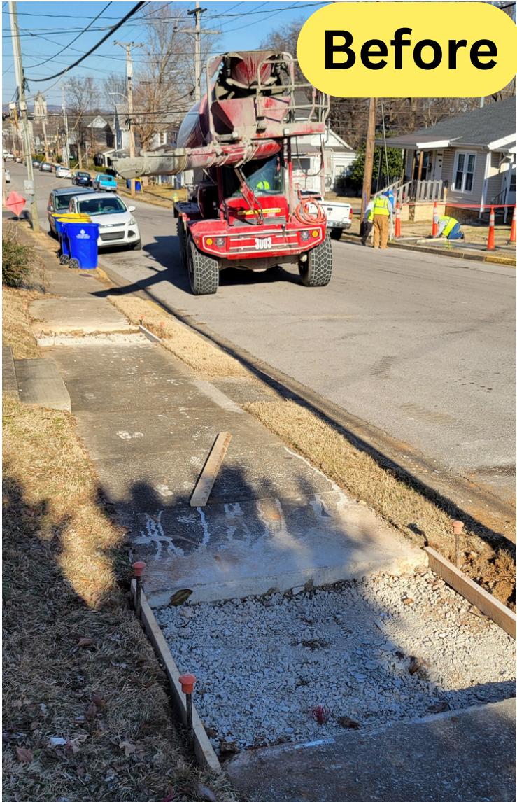
Operations Maintenance Technician III David Wilbert finishes concrete on a sidewalk repair on East 11th Avenue. Three sections were replaced along the street (28 January).
