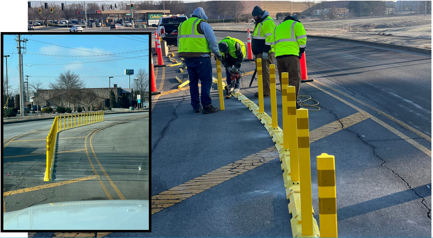
Traffic Safety Update- Our Public Works Operations crews and Planning & Design staff installed new flexible delineator posts on Ken Bale Boulevard (in front of Drake's Restaurant). The posts are designed to assist drivers in making safe turns at designated locations. Each post is plastic with reflectors and costs $53.00. (9 January)
