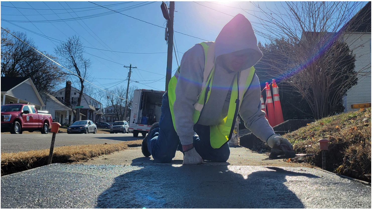
Operations Maintenance Technician III David Wilbert finishes concrete on a sidewalk repair on East 11th Avenue. Three sections were replaced along the street (28 January).
