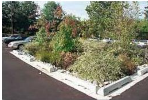
Figure PTP-10- 4 Bioretention System
