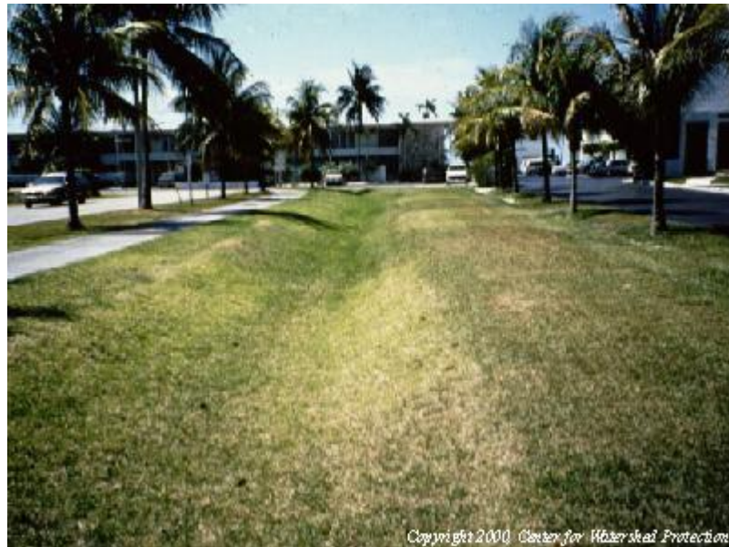
Figure PTP-02- 1 Dry Swale
